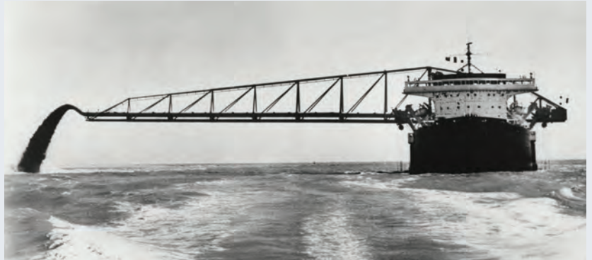
The Zulia , a large and highly effective side-casting boom and hopper dredge, was conceived, designed and built by Ludwig. Created to deepen the entrance to Lake Maracaibo in Venezuela to open access to massive oil tankers, it removed more "spoil" in 10 days than small hopper dredges had removed in two years.
